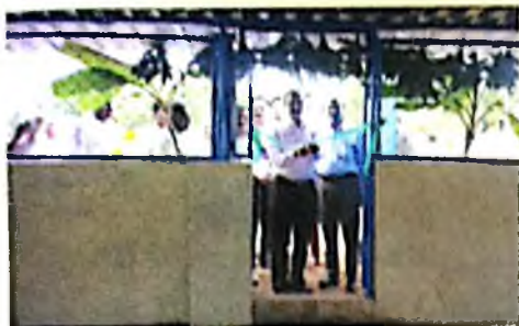
Newly constructed Sheep unit at Livestock & Research and Information Centre, Konechally. Inauguration was performed by Hon'ble Vice Chancellor.
